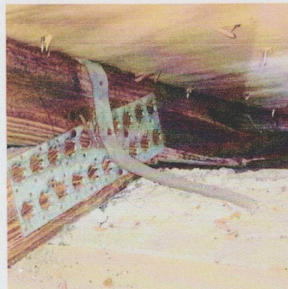
Toe Nailed (Metal connectors that do not meet the minimum requirements)
